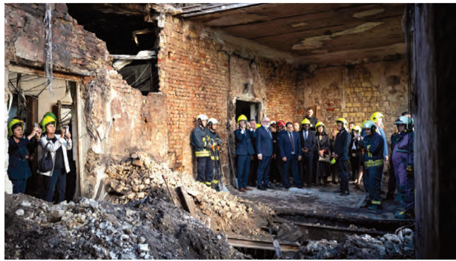
Representatives of diplomatic missions check destruction at the Cabinet of Ministers building damaged
